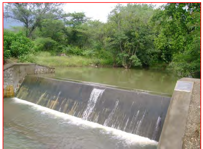
Construction of checkdam
